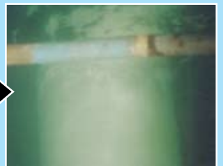
Completion of coating
