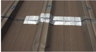
Application of Inoplast AL
