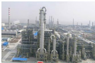
Fujian petrochemical industrial
