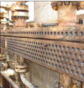
FinFan cooler before a maintenance
