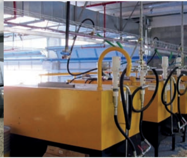
Pump room with PumpMaster 4 pumps.
