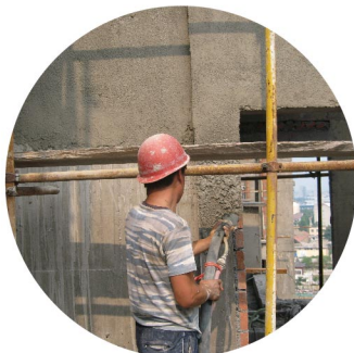
Exterior mortar spraying
