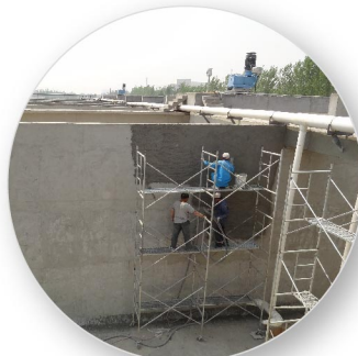
Waterproof mortar spraying
