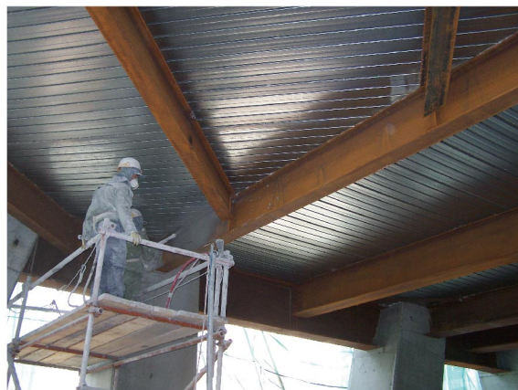
Fireproof mortar spraying
