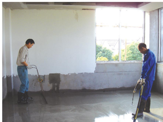
Self levelling floor screed
