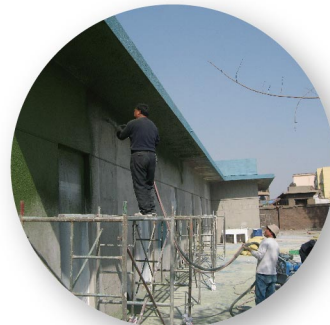
Decoration mortar spraying
