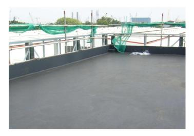
TamSeal 23 is a "coal tar free" liquid applied, single compound based on bitumen modified, polyurethane waterproofing membrane. It cures by reaction with atmospheric moisture to give a continuous seamless film which is rubbery, elastic and tough resilient film.
