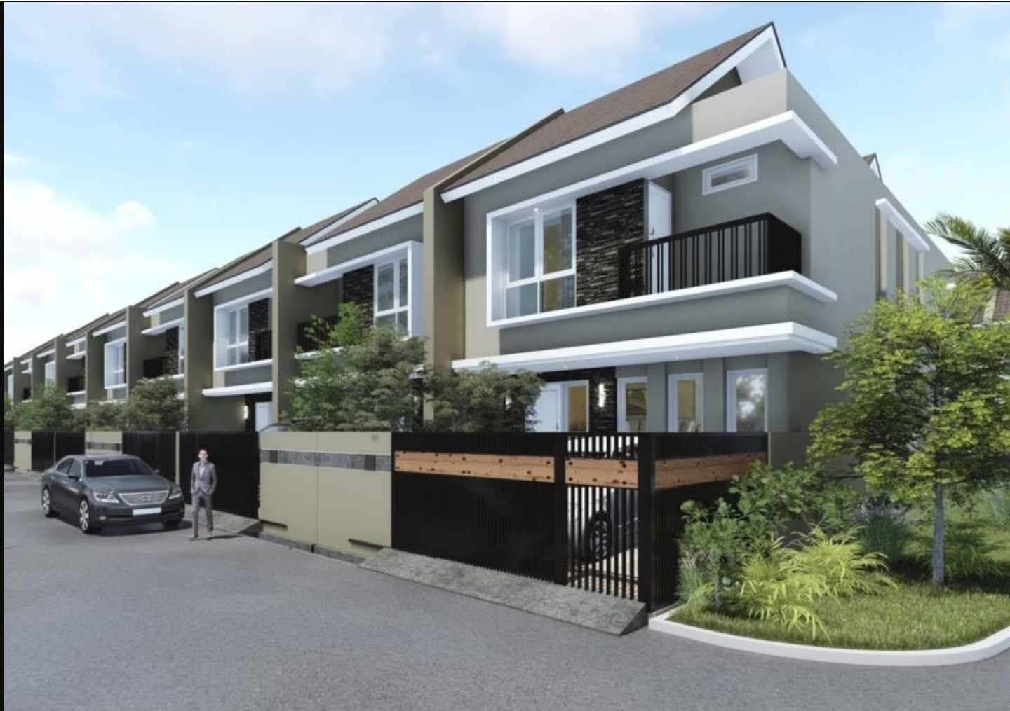
Gading Kenten Residence - Palembang
