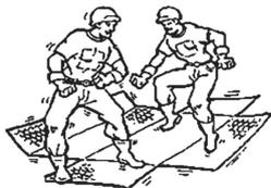
Undo the bundle and unfold each gabion over a hard flat surface.
