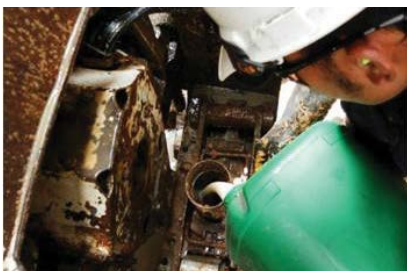
Pouring STICK UP into the rod string.
