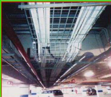
CABLE LADDER CAGE (BRC)
