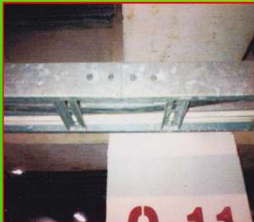
CABLE LADDER CAGE (BRC)
