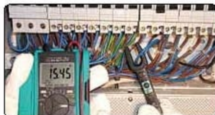
Measuring current in a Switchboard
